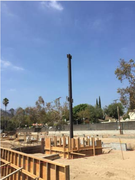
Fremont Elementary School
