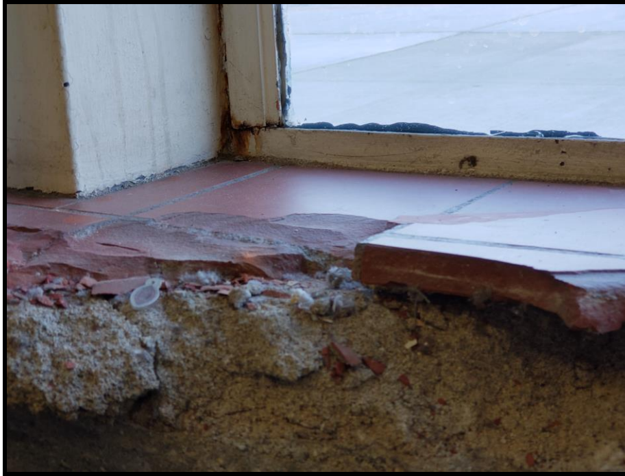
Photo #5 – Light rust at window
